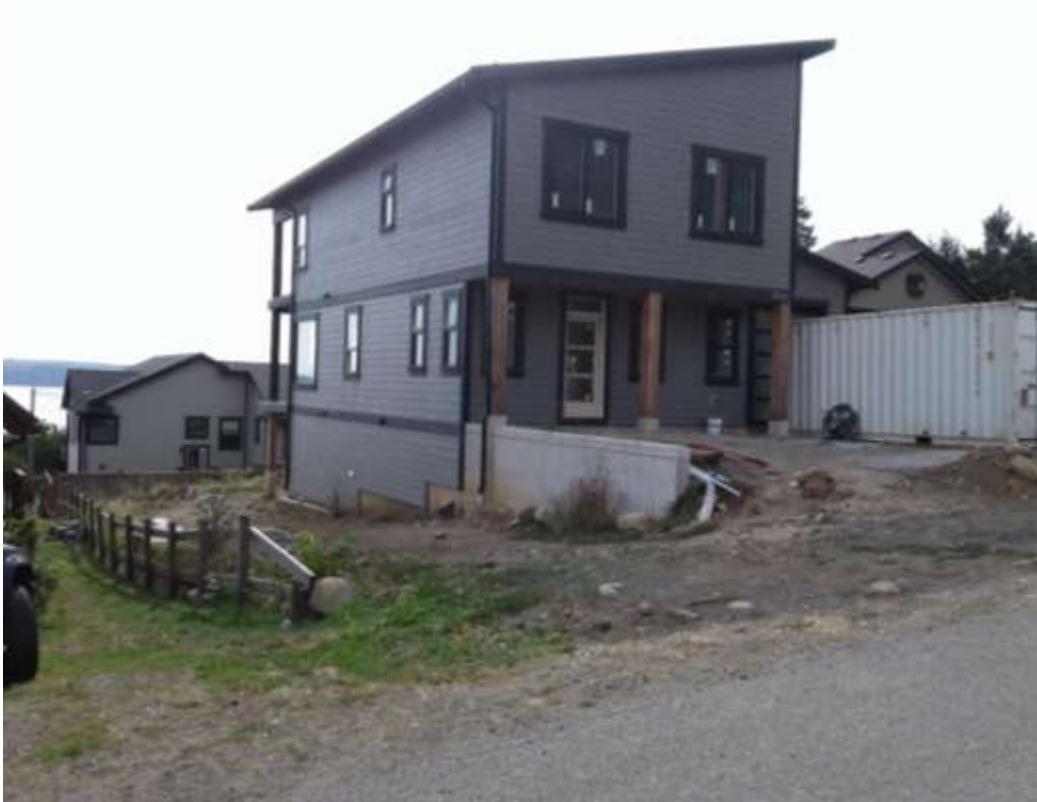
Figure 3: Subject Property Where Retaining Walls are Proposed to Surround the Backyard
